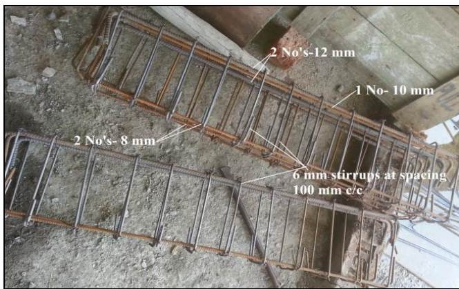
Fig 4.2 Reinforcing bars and stirrups
