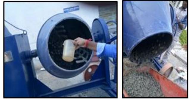
Fig. 4.2 Mixing of geopolymer concrete
