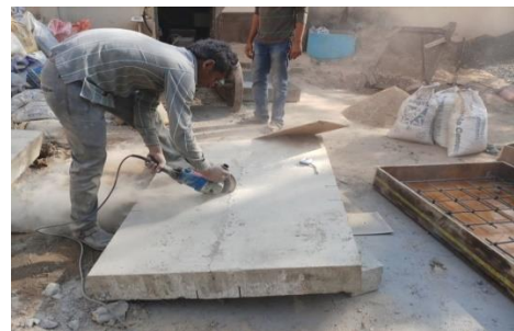
Figure: 7 Cutting of concrete
