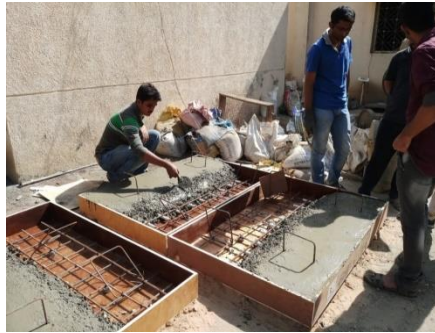
Figure 3: half casted of slab
