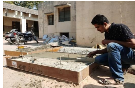
Figure 6 :fresh concrete on old concrete
