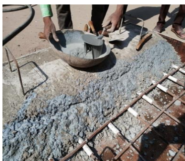
Figure 5: applying the bonding agents
