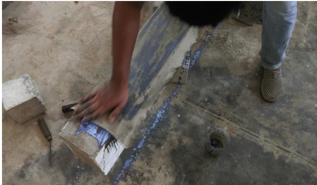
Fig 5: Fixing the basalt mesh over the beam using epoxy resin
