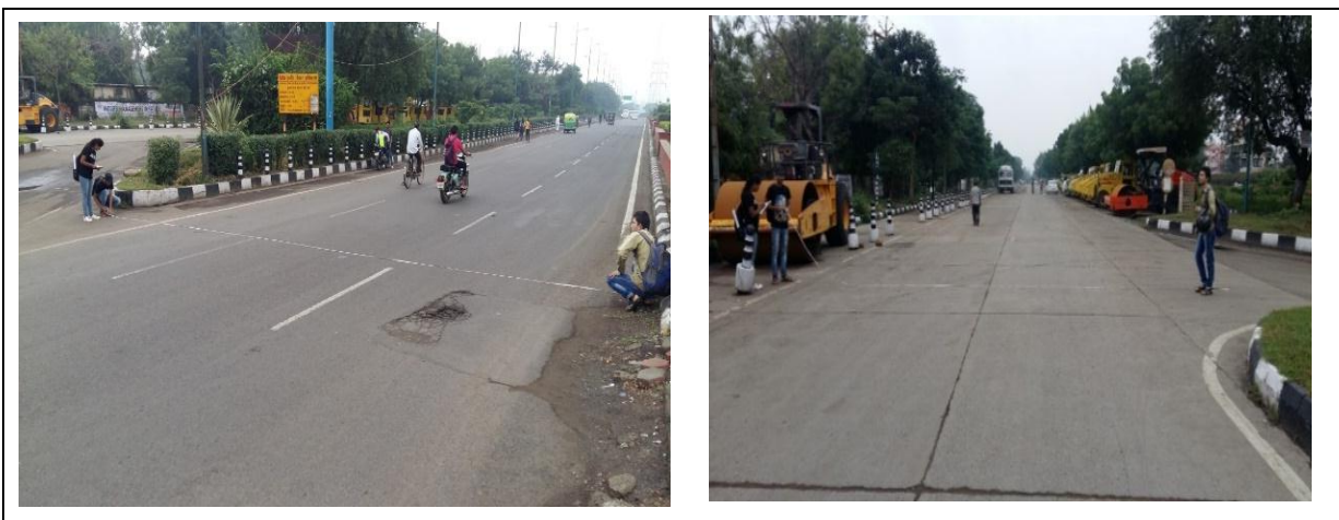
Fig.1: Measuring road width at Vijay Nagar
