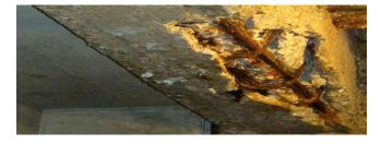
Fig -1: corroded steel embedded in concrete
