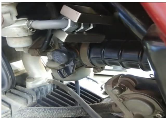
Fig- 2: Installation of Magnets on fuel line
