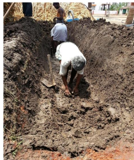
Fig -4 Digging of Bio Digester.
