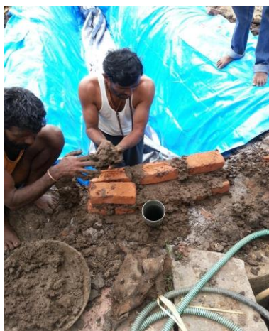
Fig -5 Installing inlet chamber
