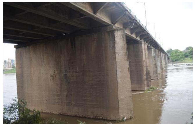
Image-1: General view of Mundhwa Bridge across Mula-Mutha river
