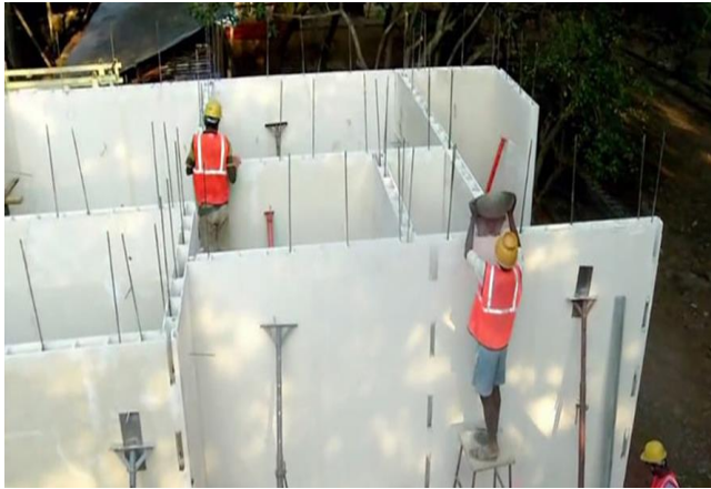
Fig -6: Construction carried out using GFRG wall panels
