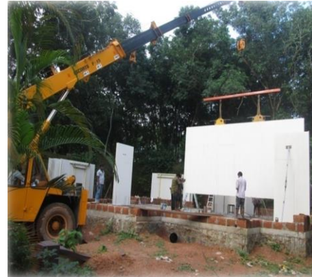
Fig- 10: Installation process
