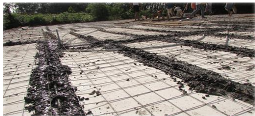
Fig - 14 : Reinforcement on slab
