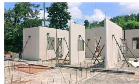
Fig- 11: supports provided for GFRG panel
