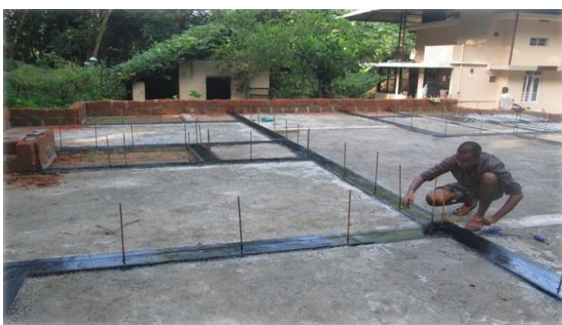
Fig- 9 : Starter bars in foundation
