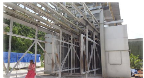
Fig- 6 : Dryer chamber
