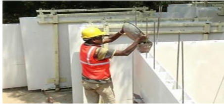
Fig - 12: Concrete filling
