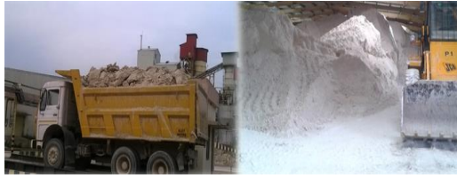
Fig - 1: Gypsum handling
