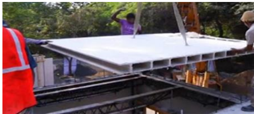
Fig- 13: Roof placing
