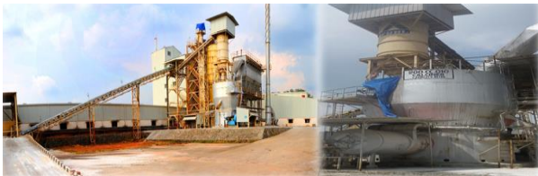
Fig- 2 : Calciner Plant
