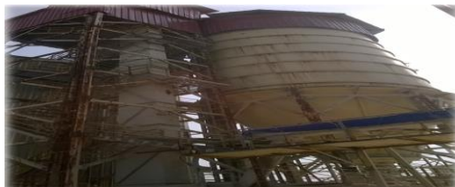
Fig - 3: Plaster Handling
