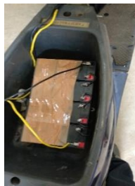
Fig 8-battery placed under the seat
