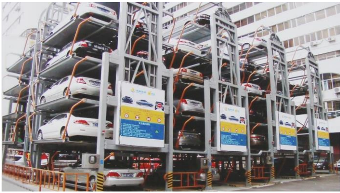
Figure 1 vertical rotary automatic car parking
