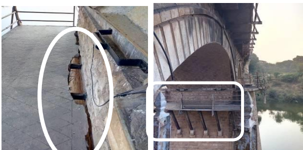
Fig11:- Gallery of bridge
