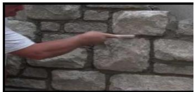
Fig4:- Mortar joint in stone masonry
