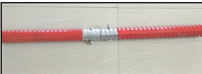
Fig-14: By Single Rod double nut method
