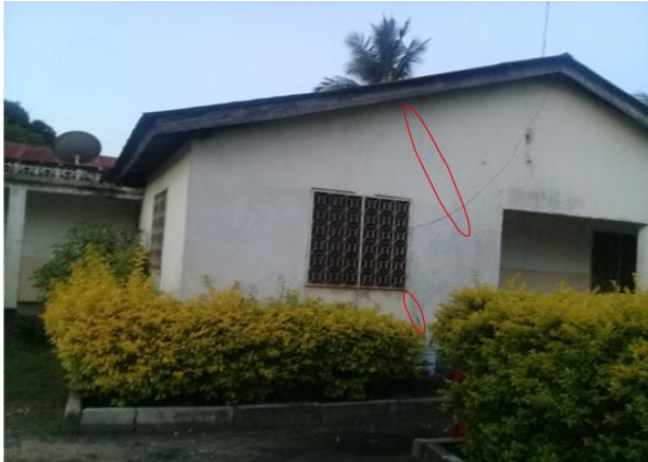
Figures 33: Poor Landscape Architecture Providing Flowers Close to External Walls Source: 2018 Field Survey in Mbweni-Dar es Salaam
