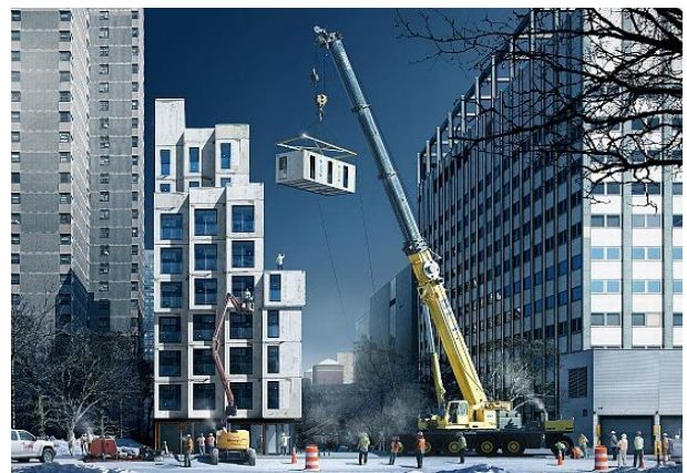
Figure 23: Modulated Factory Rooms installed on Site in New York Source: Cohen 2016
