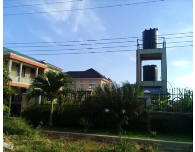
Figure 32: Good Practice: A Stand-alone Water Storage Concrete Tower Structure Source: 2018 Field Survey in Mbweni-Dar es Salaam
