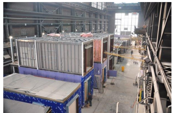
Figure 22: Modular One Bed-roomed Apartment Manufactured in a Factory Source: Cohen 2016
