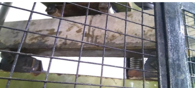
Fig -9: CB4 after testing
