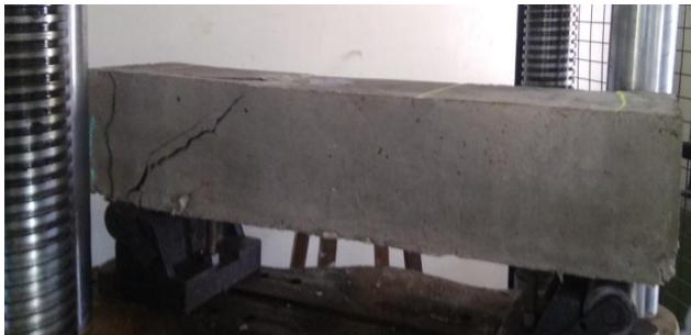
Fig -7: CB2 after testing
