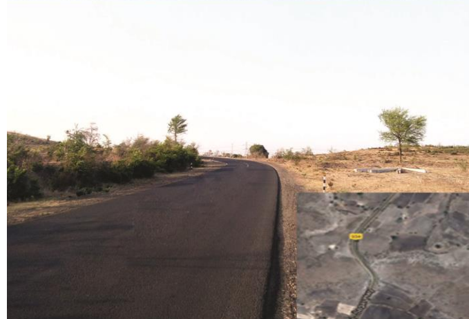
Fig 1.2 : Chhapri Turn Accident locations. Source: Site visit photography.
