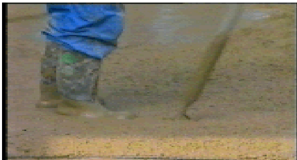
Fig-11: Concrete Vibration
