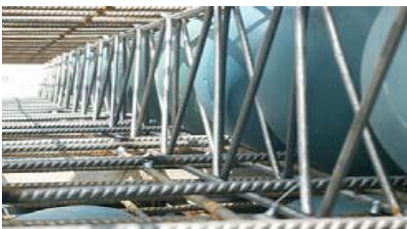
Fig- 2: Diagonal Girder
