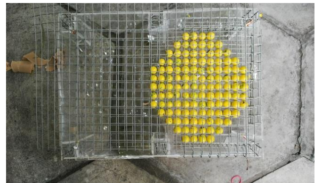
Fig-19: Provision of Top Reinforcement Meshes
