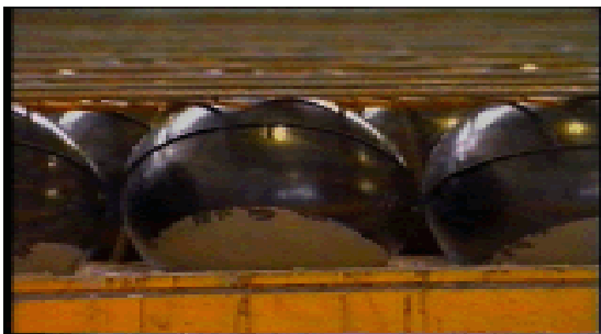
Fig- 6: Provision of Top Reinforcement
