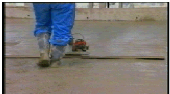
Fig-12: Concrete Slab Surface Finishing
