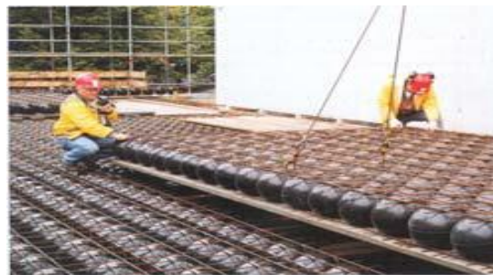
Fig- 9: Fixing Partially Manufactured Bubble Deck Slab
