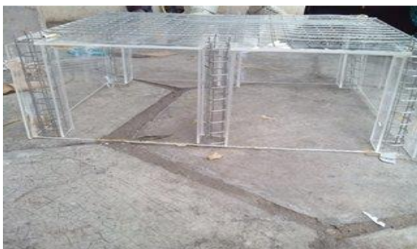
Fig-17: Column Reinforcement
