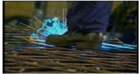
Fig-3: Bottom Reinforcement
