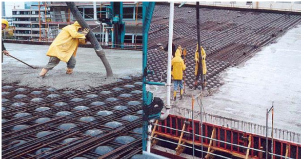
Fig-10: Slab Concreting
