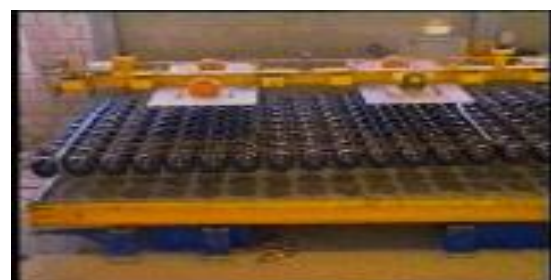
Fig- 5: Location of Hollow Spheres
