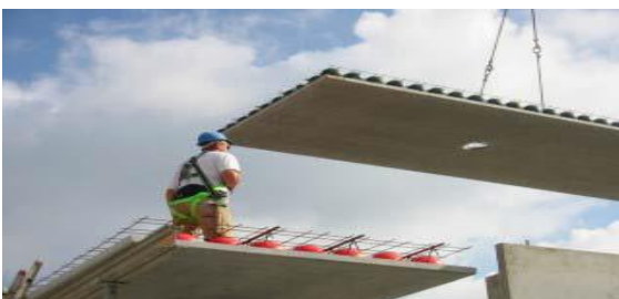
Fig- 7: Transportation of Precast Bubble Deck Slab
