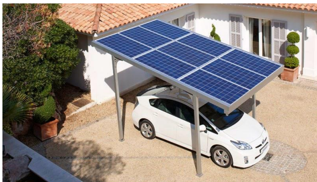
Figure 4.1 Residential charging station
