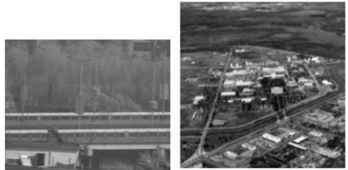
Fig -1. Bridge and Aerial view images
