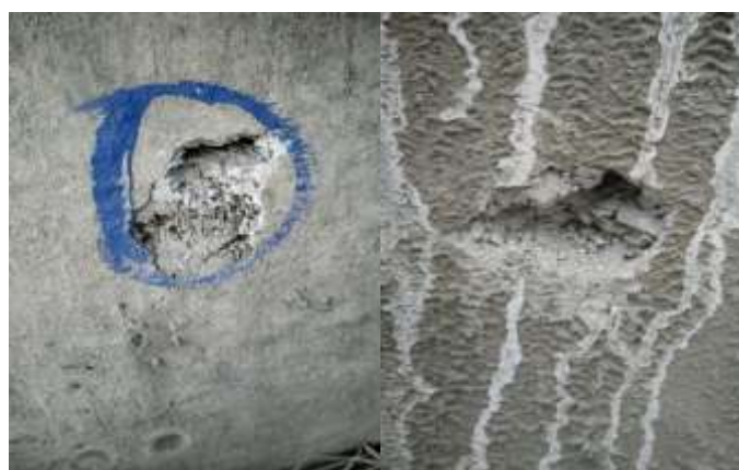
Fig -5: Pot holes Observed
