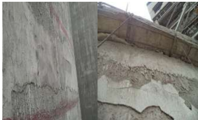
Fig -4: Hand patching and Honey combing of Concrete
