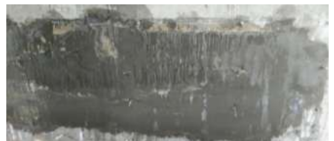
Fig -2: Curing of Repaired Patch (Final Finished Stage)
