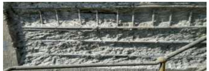
Fig -1: Distressed Concrete Chipping (Initial Repair Stage)
