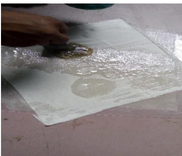
Fig - 4: First layer of reinforcement
