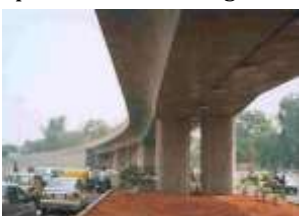
Fig -4: Kalkaji Flyover.
