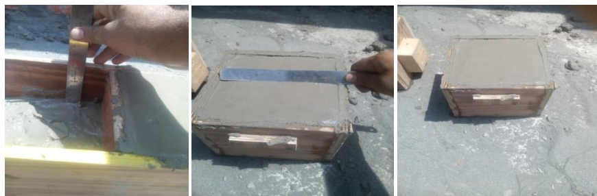
FIG.2 PROCESS OF CUBES CASTIG.
