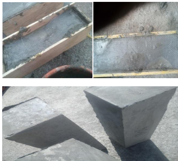
FIG 6: - RETROFITTING AND REINFORCED DETAILING OF THE BEAM.
