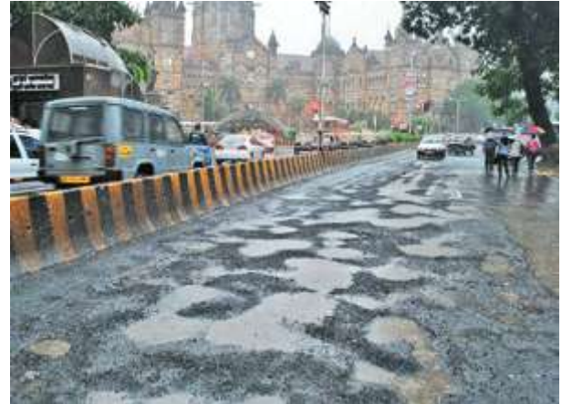
Fig 1: States of streets with Potholes
