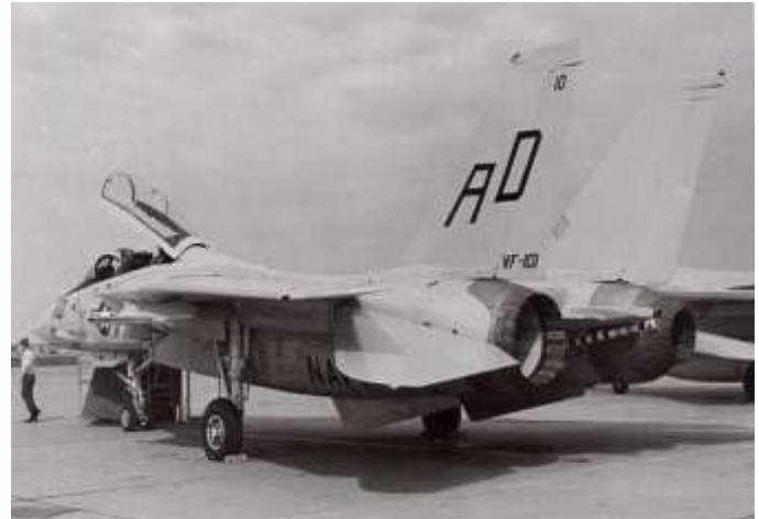
Fig -6: F-14 Tomcat-one of the first aircraft to use carbon composites
