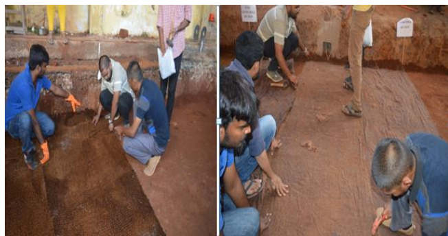
Fig-8: Installation of Coir and Jute Geo-textiles
