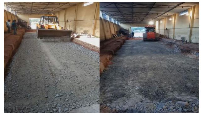
Fig-10: Spreading and Compaction of GSB material
