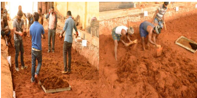
Fig-7: Spreading and Mixing of Fibers
