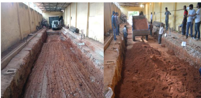
Fig-6: Excavation and Filling of Soil in test track
