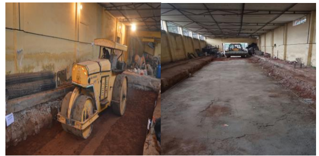
Fig-9: Compaction using Roller and finished surface
