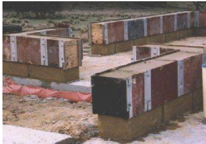
Fig - 4: Sample partition wall using cast earth and laterite
