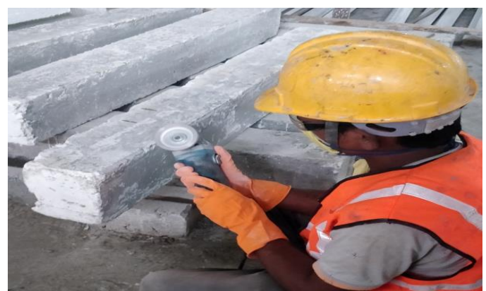
FIG-2: GRINDING TOP AND SIDE SURFACE OF BEAM
