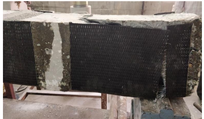
FIG-8: Failure mode of strengthened beam
