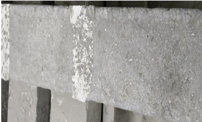
FIG-3: BEAM SURFACE AFTER GRINDING
