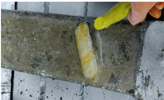
FIG-4: APPLICATION OF EPOXY AND HARDENER ON THE BEAM
