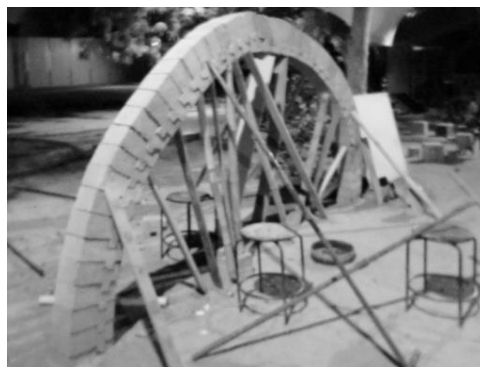
Figure 3: papercrete interlocking arch [10]
