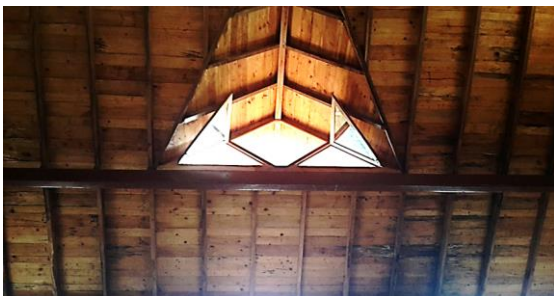
Image 12 View of the Dormer window
