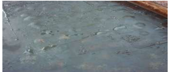
Fig. 10: Blistering of Fluid Membrane
