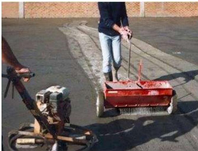
Fig. 25: Crystalline Waterproofing by Dry Shake Application Method
