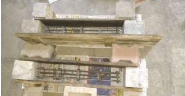
Placing of the cage in the mould
