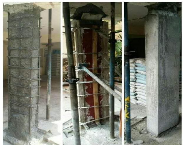
BREAKING SHUTTERING MICRO CONCRETE
