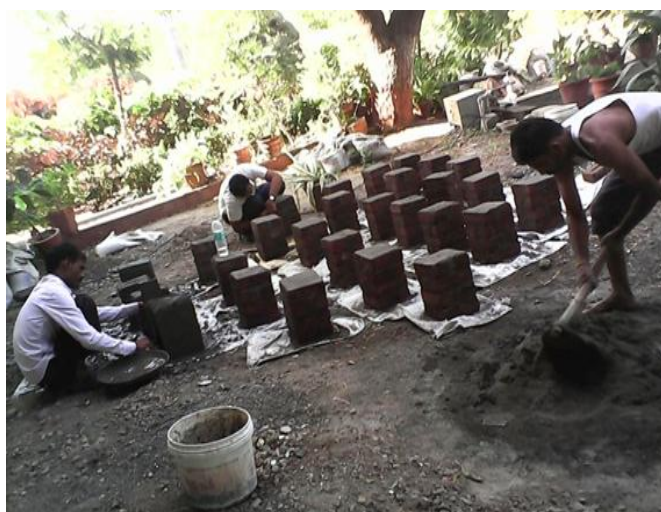
Fig 1). CASTING OF BRICK COLUMN
