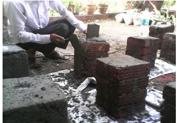
Fig 2). PLASTERING TO FERROCEMENT
