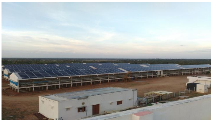
Fig 3- Solar Heating System[7]
