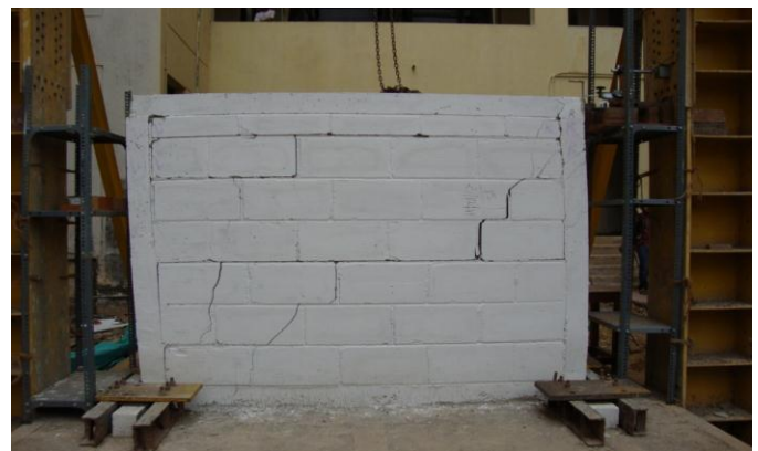
Figure 12: Crack developed at 13 th cycle loading
