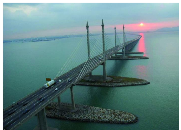
Fig - 1: View of Penang (I) bridge in Malaysia (source: Hendy, C. R. Highway &Transport Atkin)
