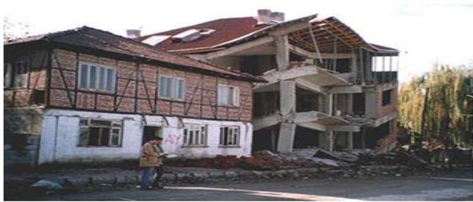
Fig -2: Dhajji-Dewari surviving October 2005 earthquake.
