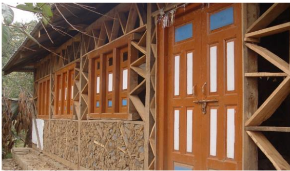
Fig -3: Dhajji-Dewari house under construction.
