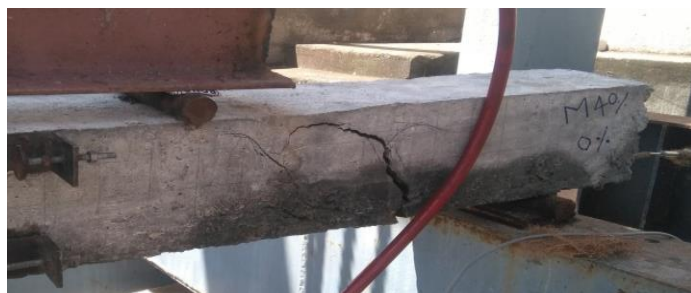
Fig 4.9. Crack profile for RC beam with 0% lapping
