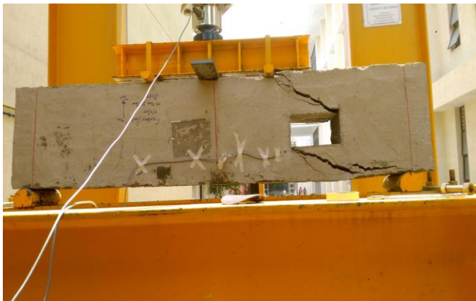
Fig 5 - The failure of beam after the test
