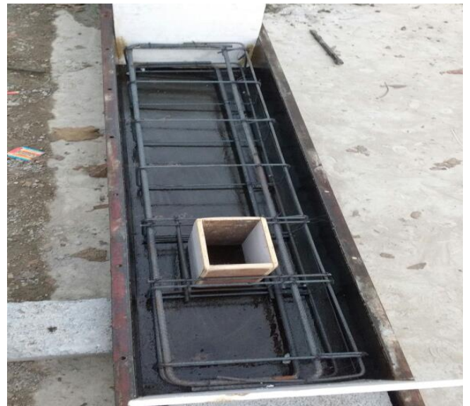
Fig 3 – Casting of beam
