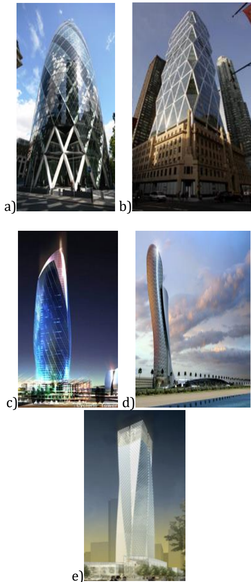
Fig. 1. Diagrid buildings (a) Swiss Re in London (b) Hearst Tower in New York (c) Cyclone Tower in Asan (Korea) (d) Capital Gate Tower in Abu Dhabi and (e) Jinling Tower in china.(ref-paresh.v.patel dec.2013)
