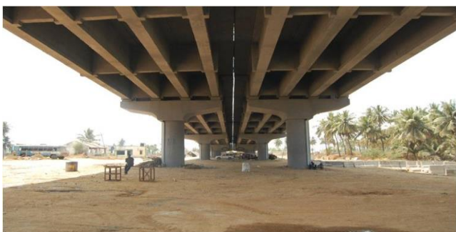
Figure 1.1: Typical I-girder bridge
