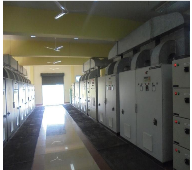
Fig-4: GEC [Grid Export Condition] inverter
