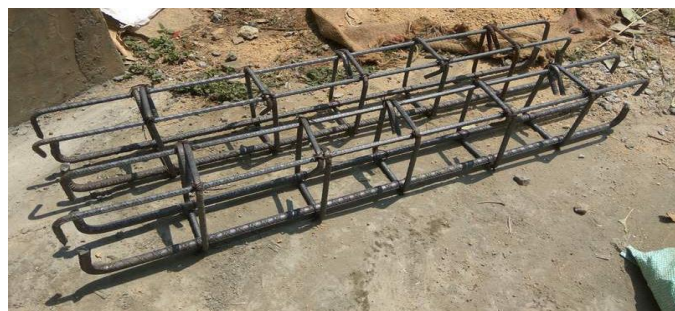
Fig -4: Reinforcement Bars for beam
