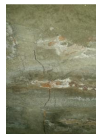
Splitting Failure of 6-Layer Red Brick Prism
