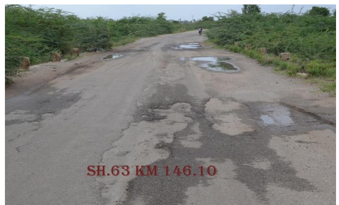
Fig- 4: Existing condition of road at Ch.146.10 (Reconstruction)
