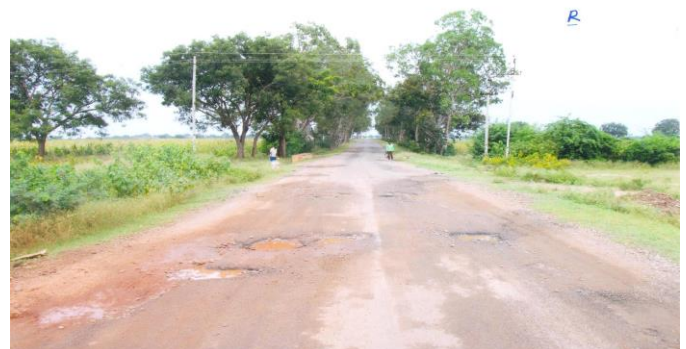
Fig-3: Existing condition of road at Ch.18.40 (Reconstruction)
