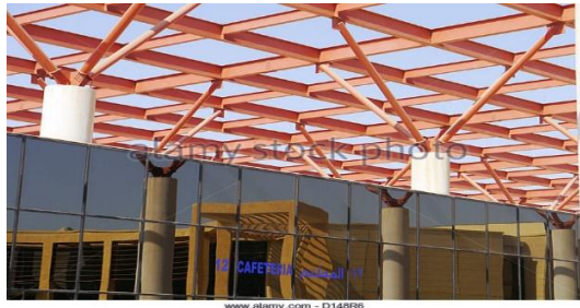
Fig:2 Typical Figure of Oblique Column
