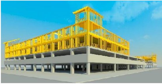
Fig:1: Typical Figure of Podium structure
