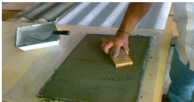
Fig -2 Placing materials to mould
